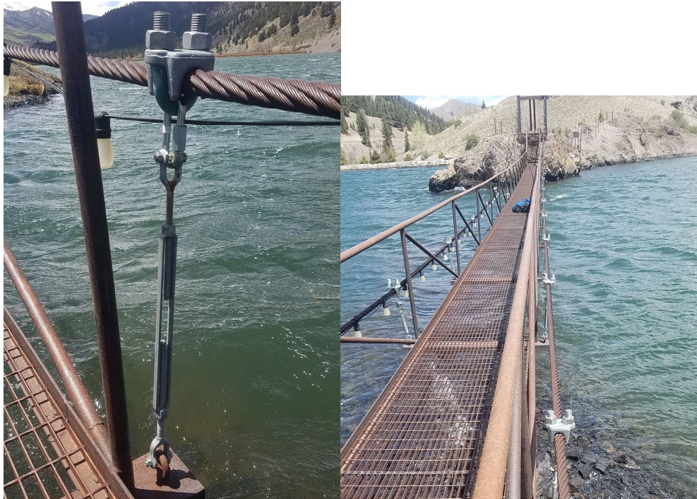
New Configured Suspender and View along East Main Cable
