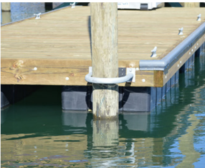
Floating dock on pier
