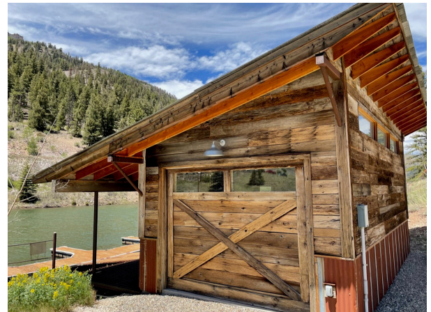
Existing Boat House
